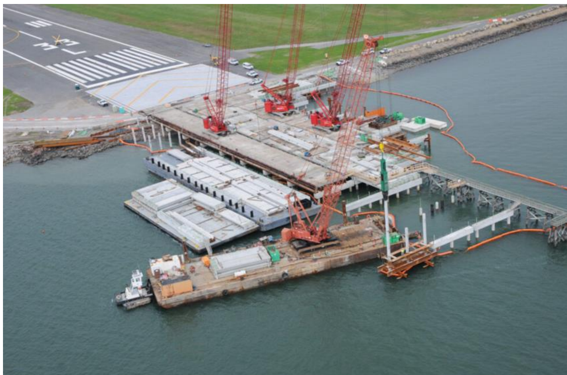
Figure 16: Typical Deck on Piers – Boston Logan International Airport Threshold 33L RESA 13
