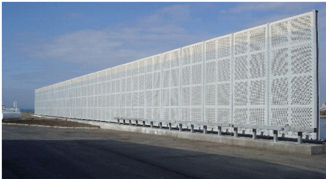
Figure 19: Existing Absorptive Sound Wall-West End of Airport
