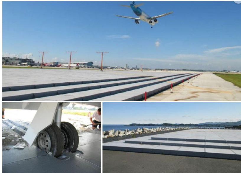
Figure 25: Runway Safe Inc. 17 EMAS Installation Examples
