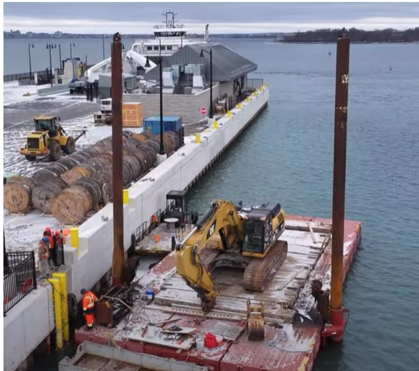
Figure 15: Typical Vertical Retaining Wall (Sheet pile) - Wolfe Island Ferry Terminal, Marysville
