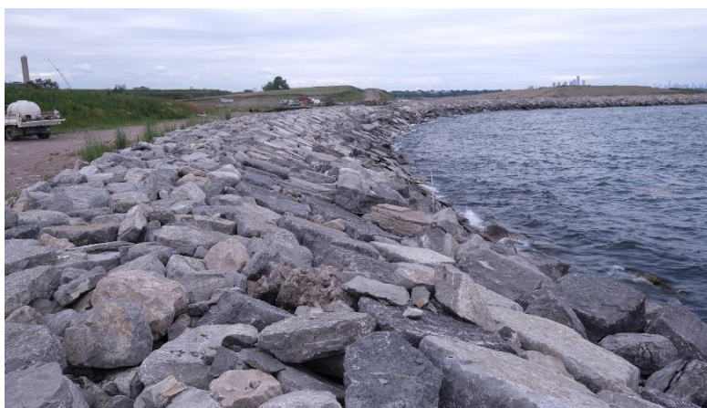
Figure 13: Typical Armour stone Breakwater/Revetment - Jim Tovey Park, Mississauga
